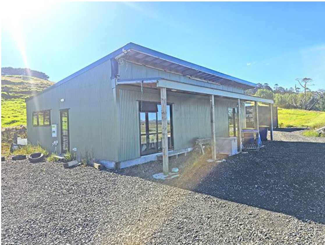
Shed from Drive, House Site elevated behind
