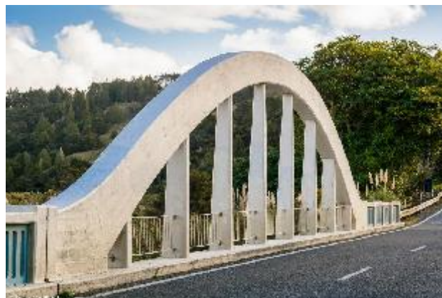
Makarau Bridge, north of Kaukapakapa
