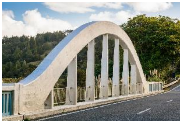
Makarau Bridge, north of Kaukapakapa
